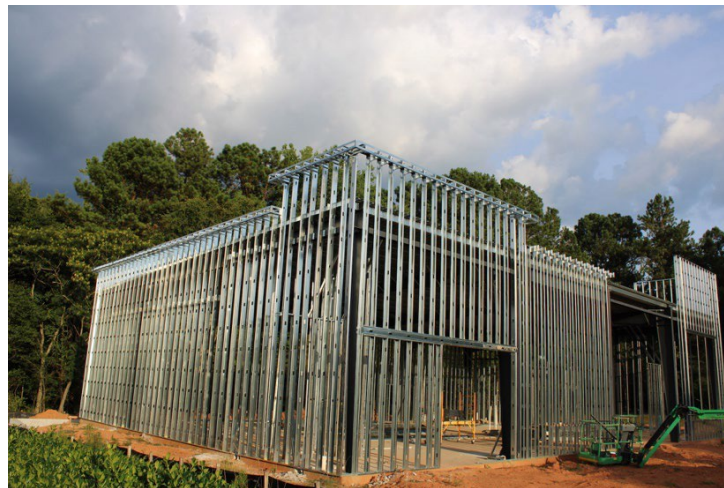
Figure 1: Cold-Formed Steel Framing Products
