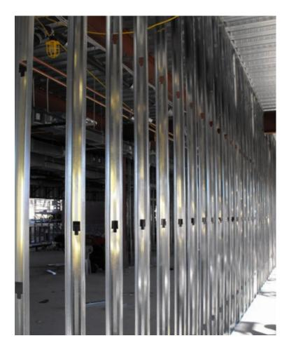
The EDGE<sup>™</sup> Steel Framing System features lightweight and high-strength steel combined with an innovative design that incorporates a closed triangular lip. This patented steel stud system provides the framer with the safest installation environment in the industry.
